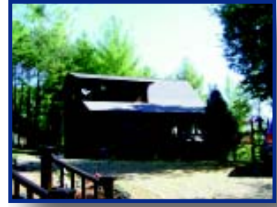
LAKEVIEW BEAR PAW HOME with 2BD/2 full baths/2 half baths, rec room, craft room and 30AMP service for RV! Intercom system, CHA, mountain and lake views. NC102213 $259,900
